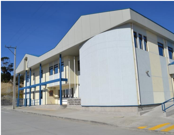
Hospital de Puerto Williams
